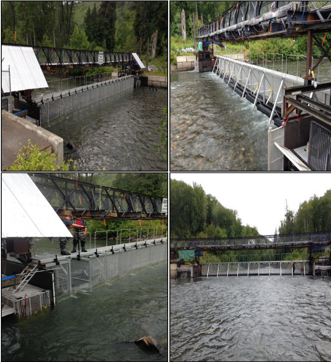
Figure 2: Photo series of the KSEF structure including new rotating fence panels, right and left bank counting stations, overhead walkway, and HDPE floats secured to the back of the panels to prevent salmon from jumping.
