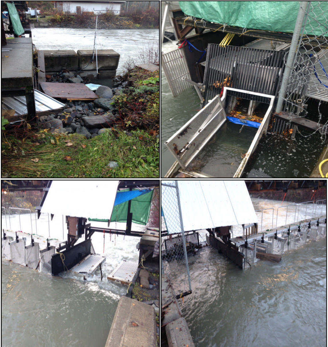
Figure 4: Photo series of the high water event and breaching of the fence on October 9 th , 2015 that disabled both the left and right bank counting boxes.
