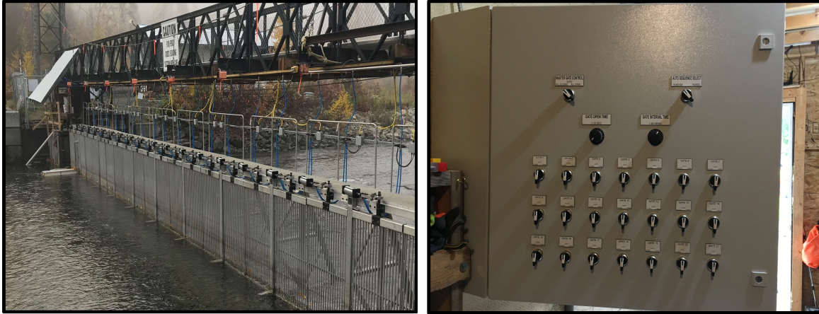
Figure 2: Photo on left shows automated panels and photo on right shows PLC panel where automation parameters can be set.
