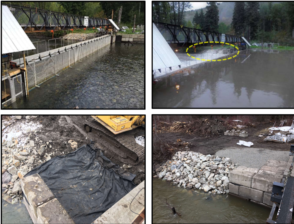
Figure 6: Photo on top left - taken during normal operating flow and photo on top right on September 11th, 2017, during extremely high flow, with yellow oval highlight right bank overflow. Photo on bottom left, right bank stabilization in process (March, 2018) and bottom right, finished work.
