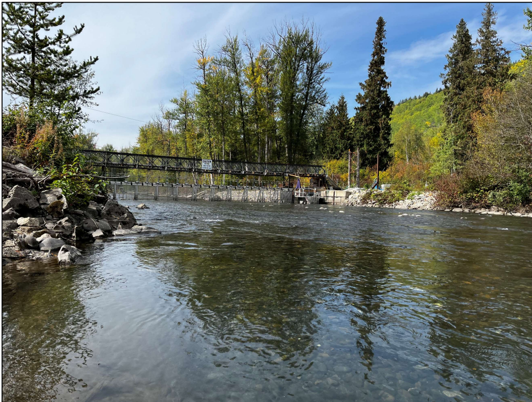
Downstream view of KSEF on September 14, 2023
