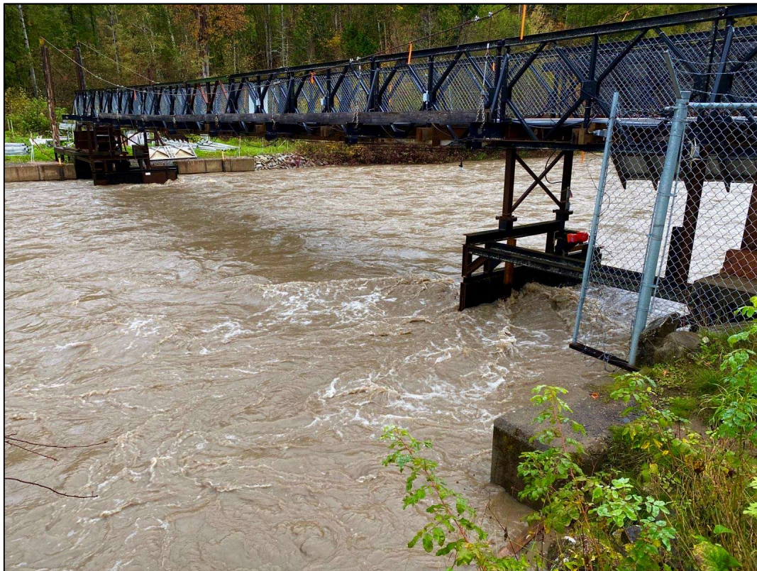
Upstream view from left bank showing fence removed. Note high water (water level was up to 1.65m even with the fence removed on Monday, September 28).
