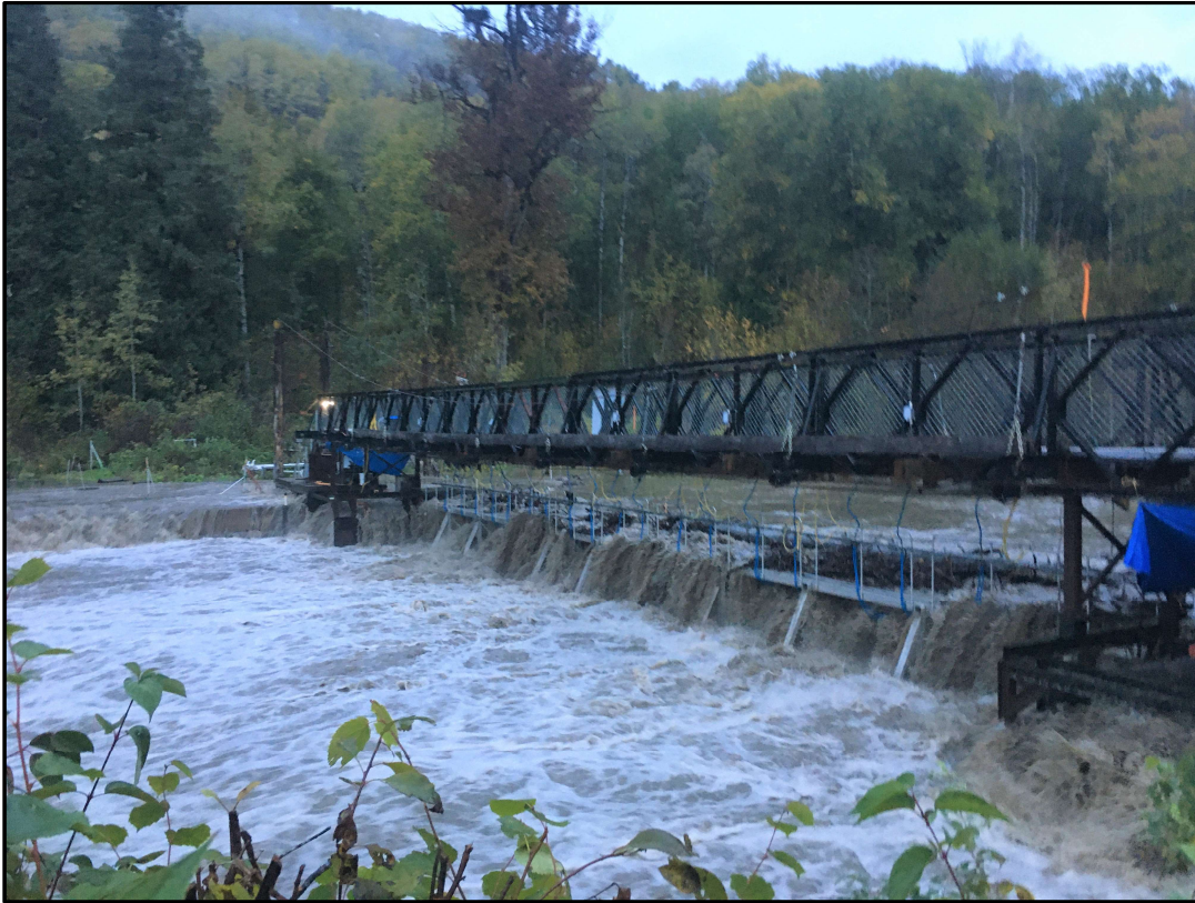
Figure 8: Photo during the night on top left shows water up to counting boxes and near to top of panels. Photo on the top right shows water and debris built up to top of panels and water spilling over right bank. Bottom photo shows view towards right bank of water overtop of sampling area on left bank.
