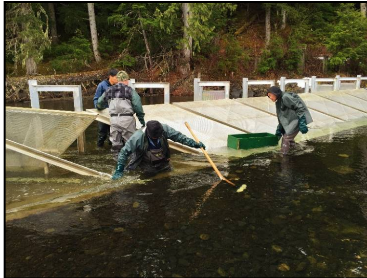
Figure 2: Photos series showing installation of KsF, including transoms (upper left), and panels (upper right)
