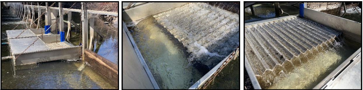
Figure 8: Photo series showing v-trough and stop-logs (left), high flow situation (middle) which needed adjustment and photo on right showing adjusted v-trough
