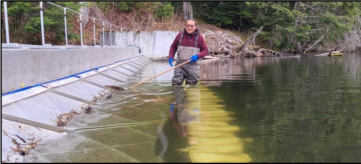
Figure 7: Photo showing GFA technician cleaning debris off panels
