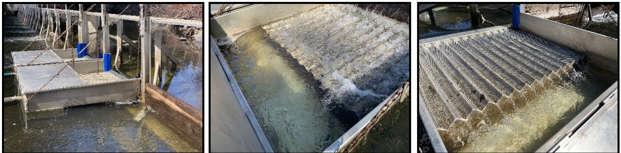
Figure 11: Photo series showing v-trough and stop-logs (left), high flow situation (middle) which needed adjustment and photo on right showing adjusted v-trough
