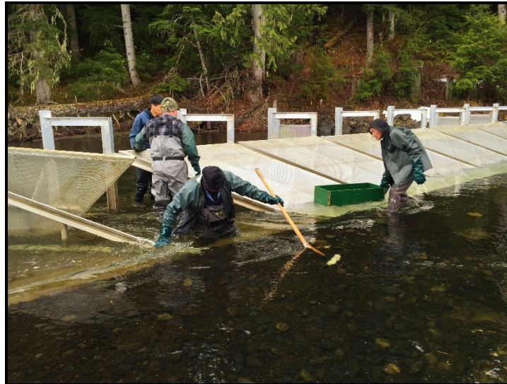
Figure 5: Photos series showing installation of KsF, including transoms (upper left), and panels (upper right)
