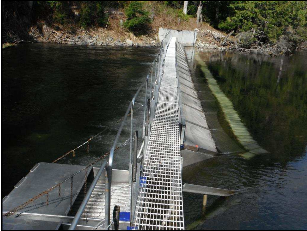
Figure 2: Completed aluminum weir installed in 2013 with new non-skid walkway and safety railings.
