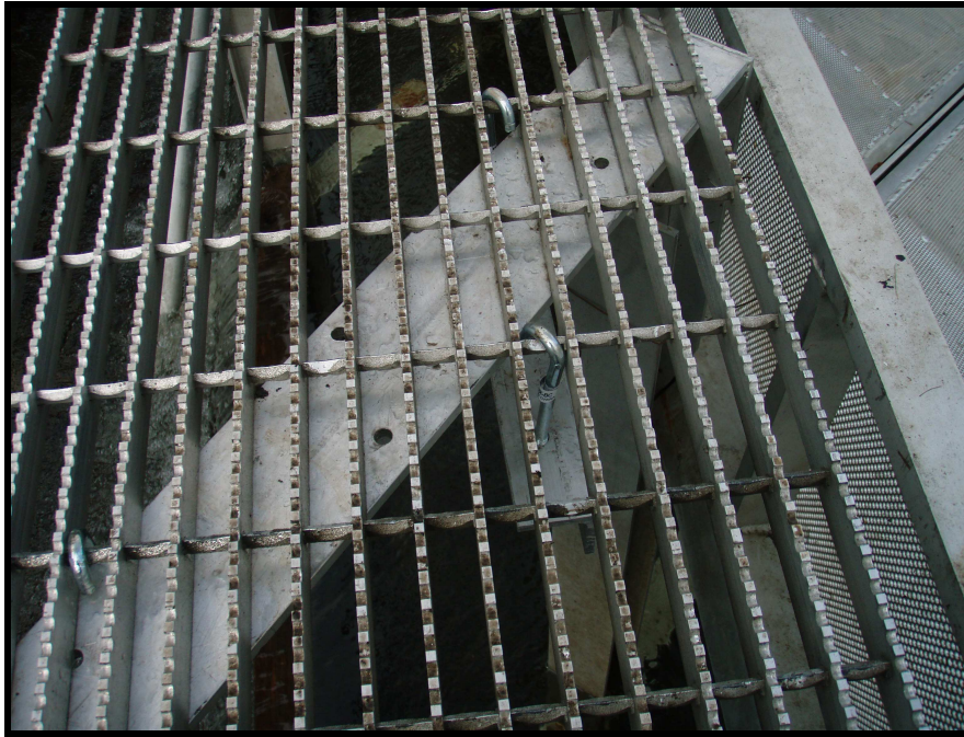
Figure 7: Aluminum walkway clamps fastened to the walkway and transoms.
